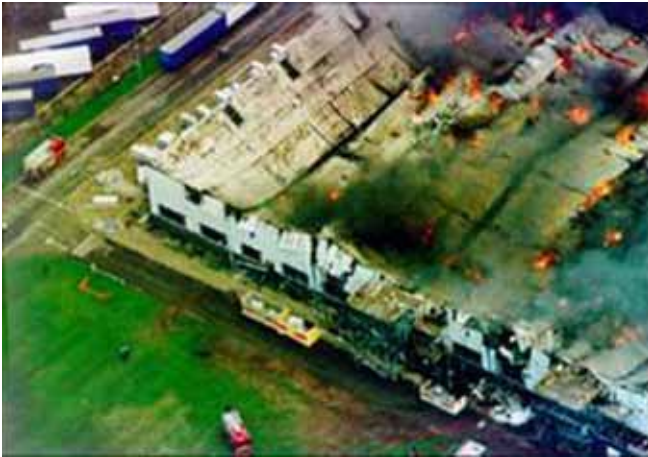
The Boots accident in Nottingham, UK. This accident was the result of flammable material being ignited by a fork lift truck.
